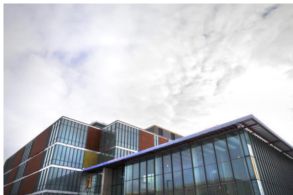
MCGS will be held in CMU's new Biosciences Building
